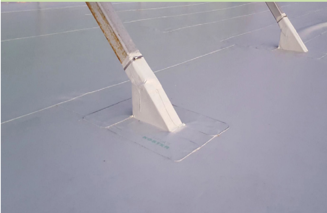
Junctions to right-angled penetrations
